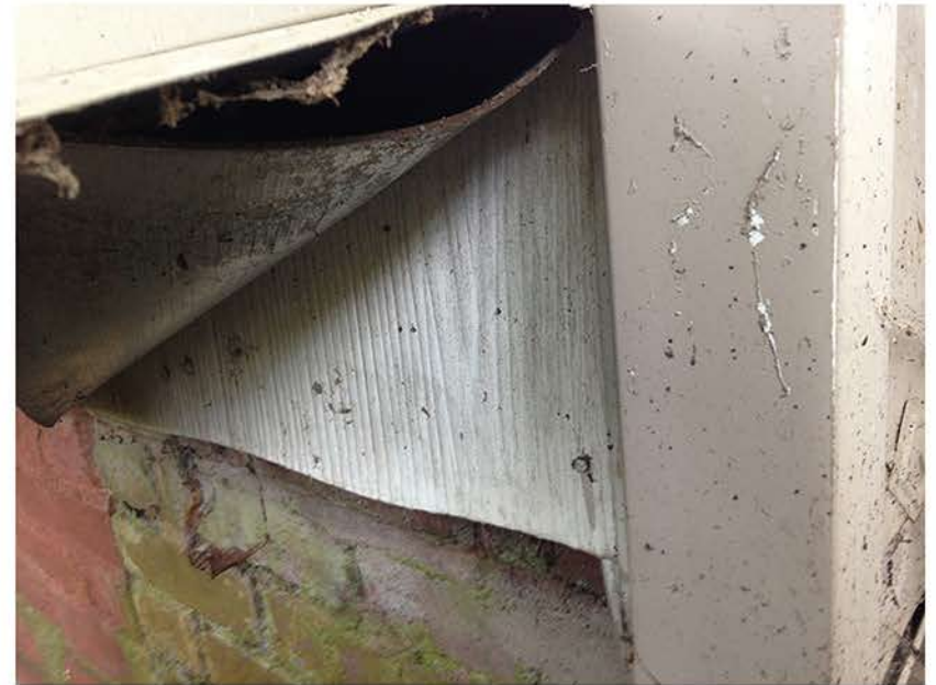
Existing masonite shown below aluminum siding
