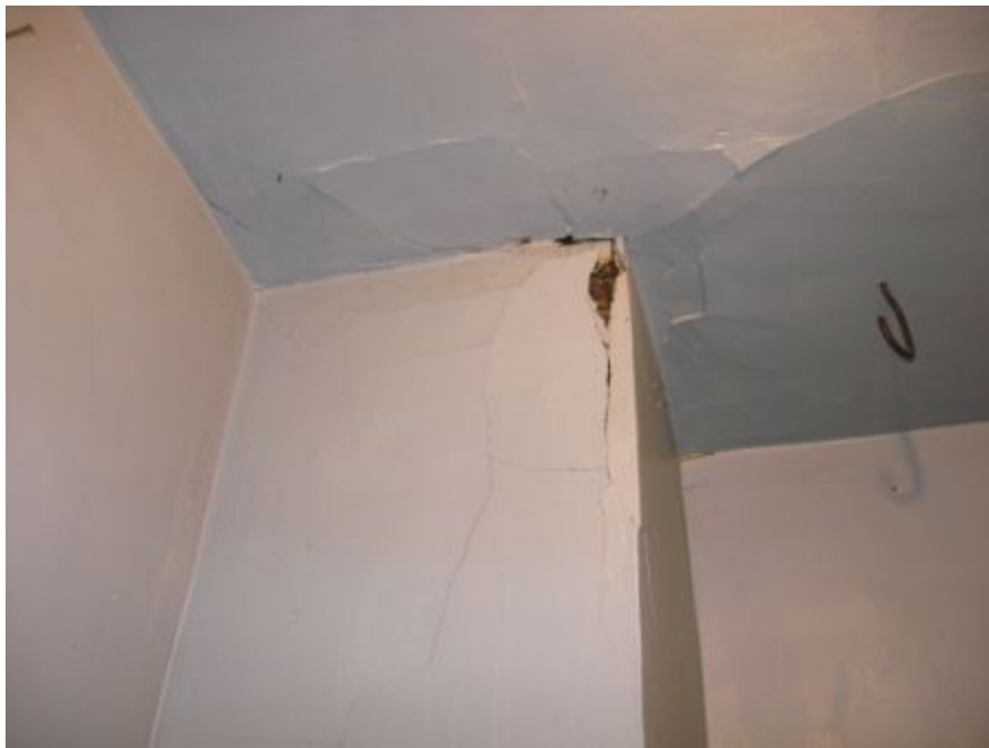
Below: Cracked Plaster, Photo 6
