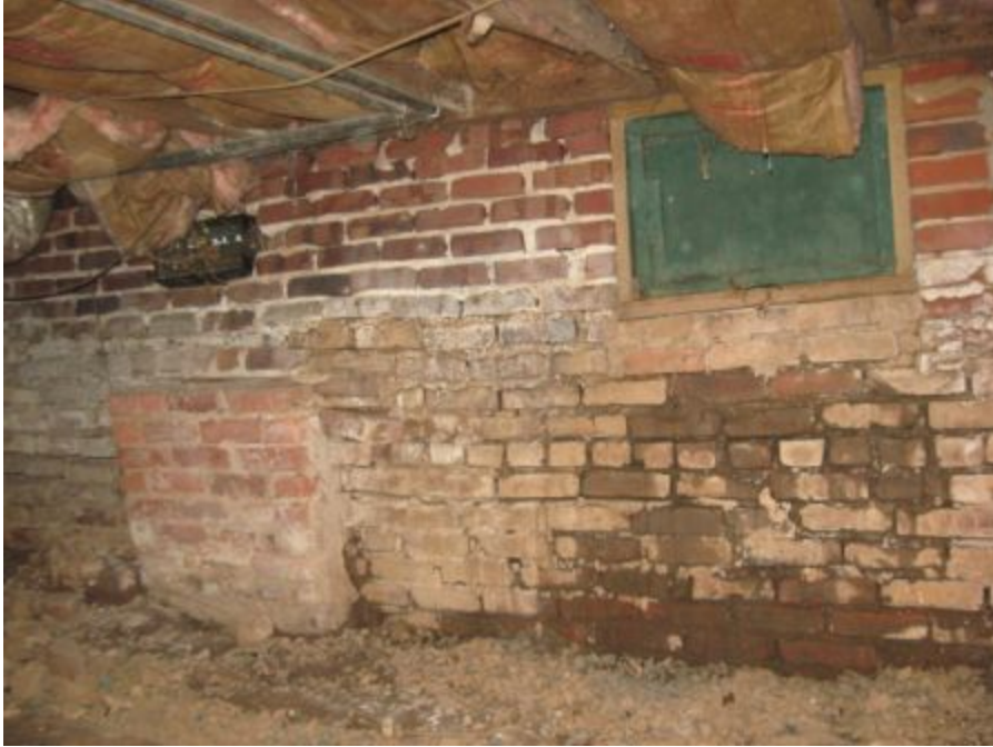
Above: Failed Masonry Curtain Wall, Photo 29
