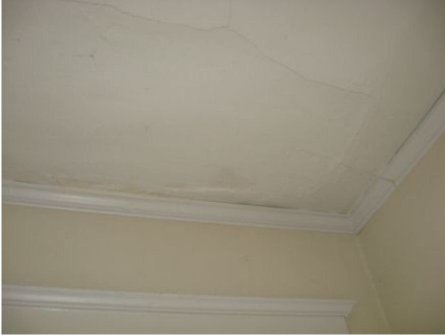
Above: Cracked Plaster, Photo 4
