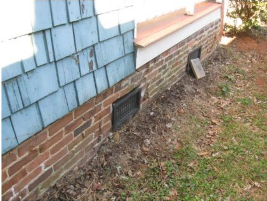
Above: Bowed Masonry Curtain Wall, Photo 18
