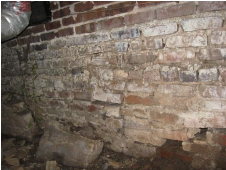
Below: Failed Masonry Curtain Wall, Photo 27
