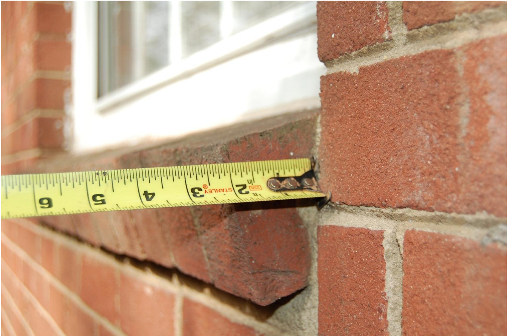
Sill protrudes 2 inches past side wall.
