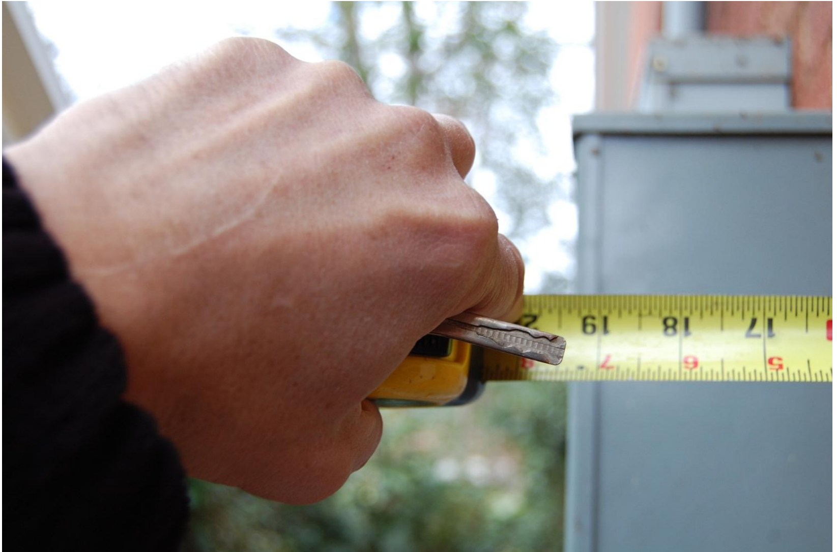
Power box and side wall extends 19 3/8 inches past addition wall.
