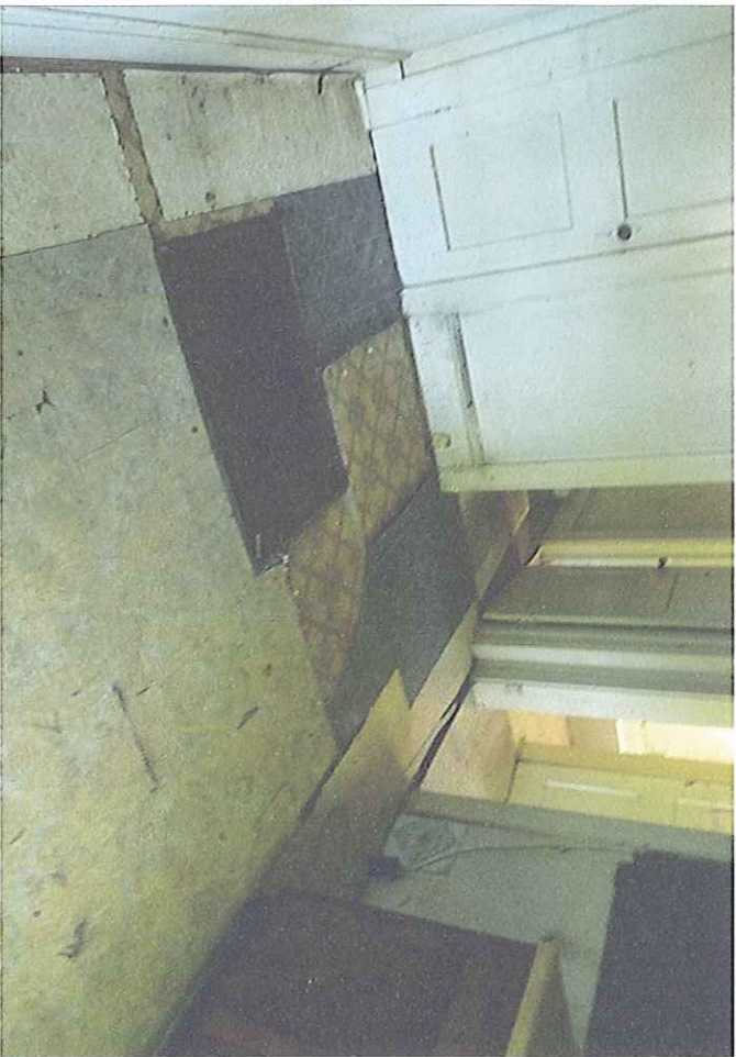
Kitchen - Sub-Floor Damage Bandsilk
