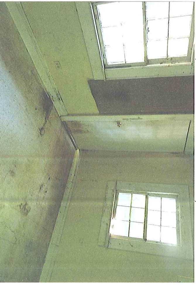
REAR ENCLOSED PORCH High moisture & Peeling STRUCTURAL Damage
