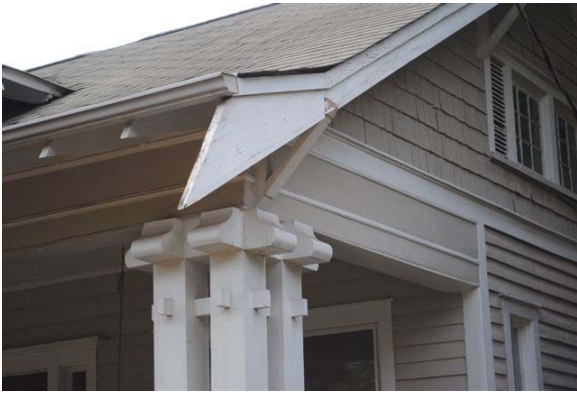
Detail at barge rafter
