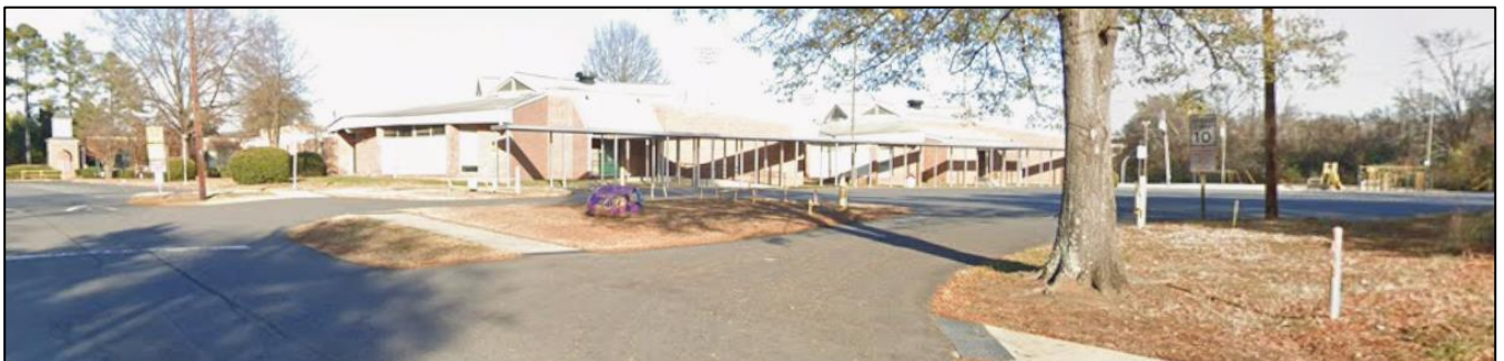
Street view of Steele Creek Elementary School to the west of the site.
