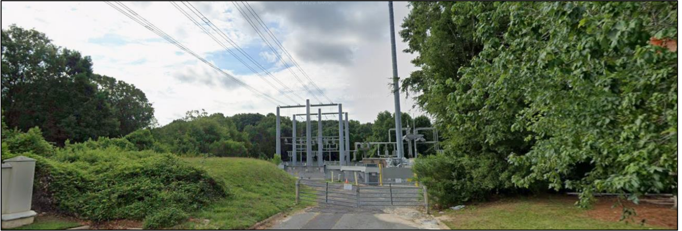
This is a street view southeast of the site and contains utility infrastructure.
