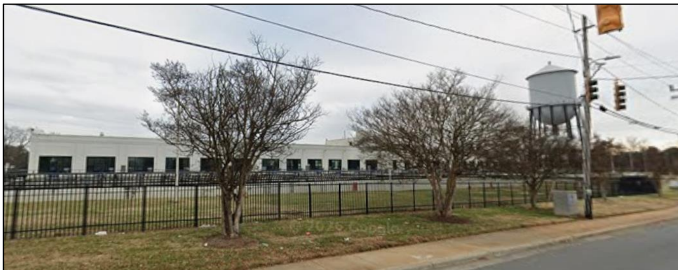
View of the Charlotte Water facility located across Beatties Ford Road from the subject site to the east.
