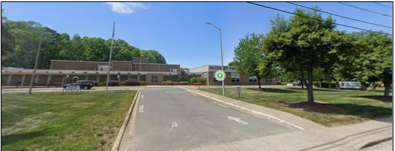
View of the McCrorey YMCA located southwest of the subject site across Beatties Ford Road. The YMCA is accessible to the proposed development via the signalized intersection of Beatties Ford Road and Capps Mine Road.
