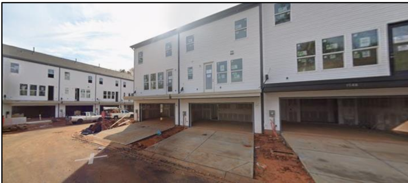
The property to the North along Blanche is developed with multi-family homes.
