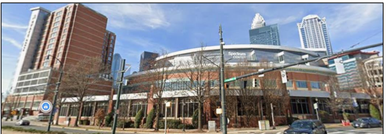
View of the site looking west from the intersection of East 5 th Street and North Caldwell Street. The existing electronic sign, located on the East Trade Street façade of the arena, is proposed to be relocated to one of three locational options, including a location on the structure near the intersection of East 5 th Street and North Caldwell Street (at the right of the image) or on North Caldwell Street (at the left of the image).
