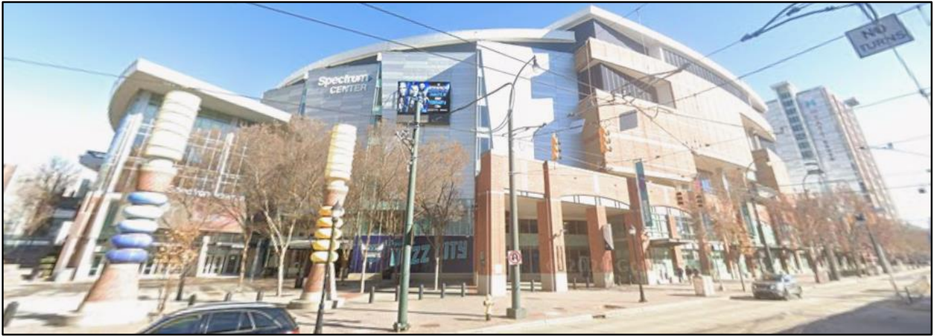
View of the site looking east from East Trade Street. The existing electronic sign, shown in the image, is proposed to be relocated to the East 5 th Street or North Caldwell Street side of the arena. A new, larger electronic sign is proposed to replace the current sign.
