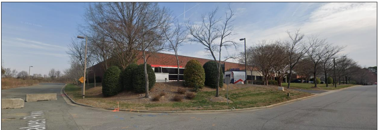
East of the site is an industrial building with some office space.
