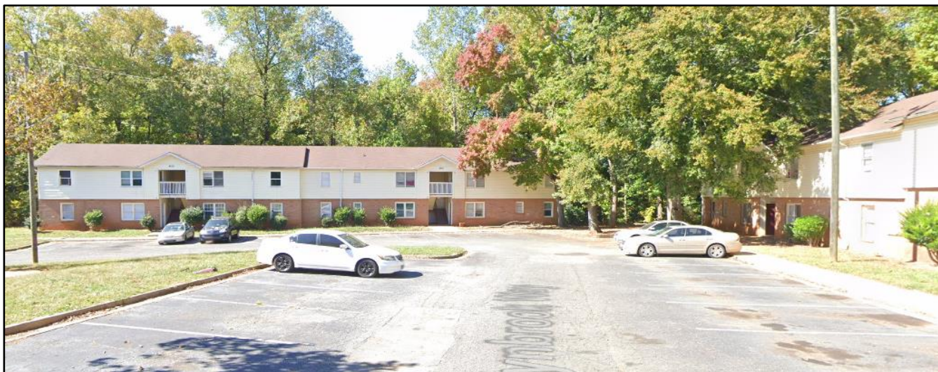
View of a the Dalecrest Multi-family development located to the east of the site zoned N2-B (Neighborhood 2-B).
