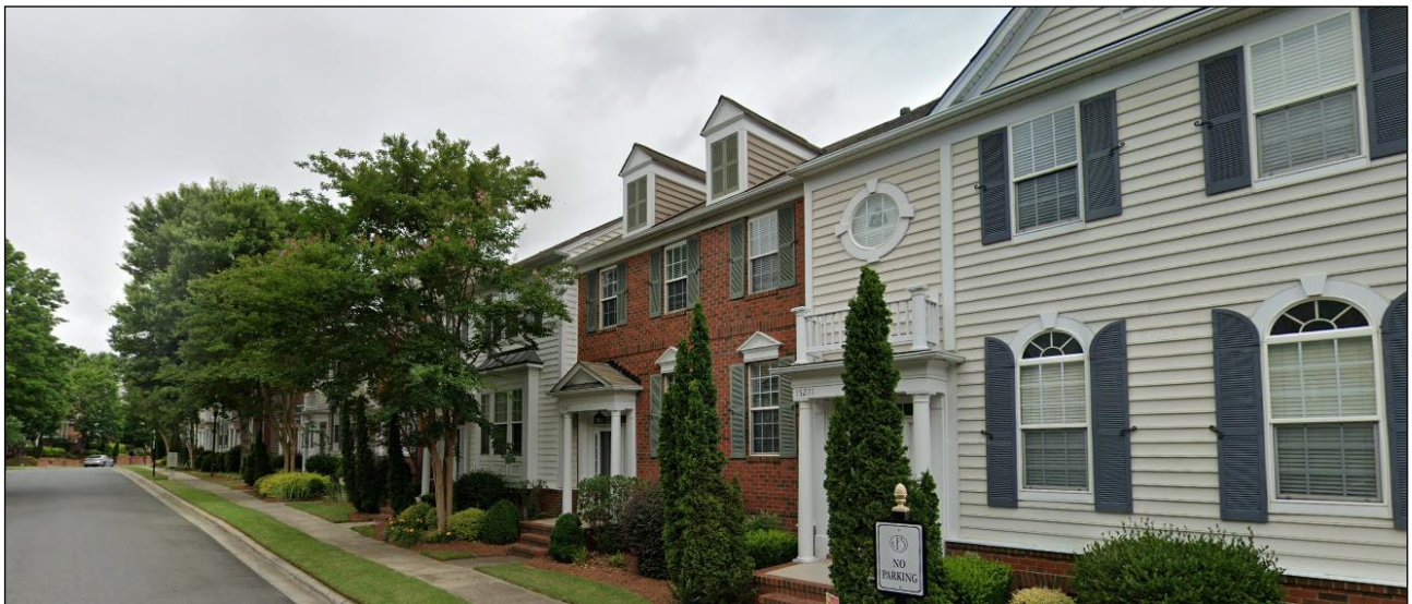
South of the site are townhomes.
