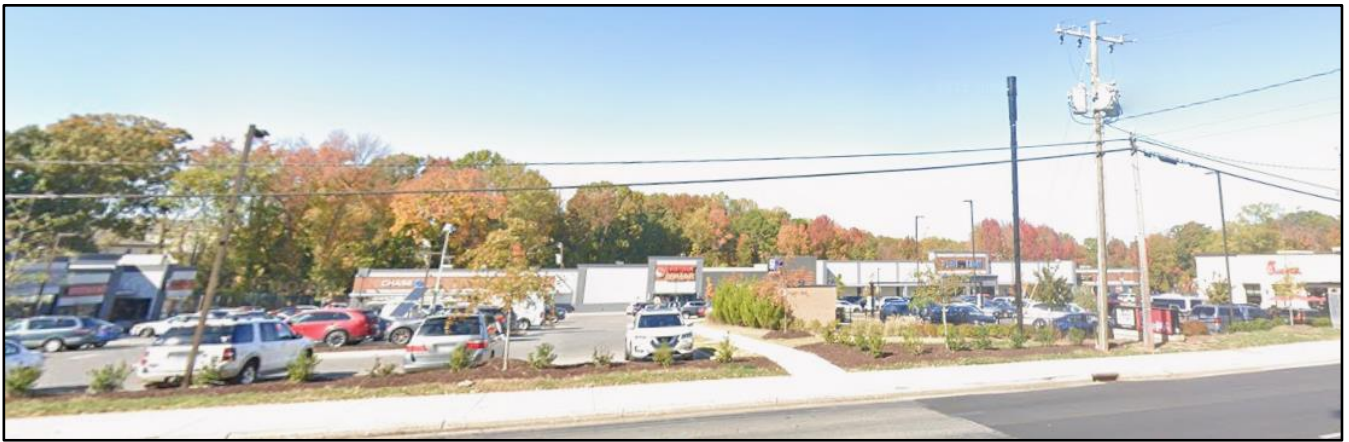
View of the Wendover Plaza Shopping Center, which provides daily needs such as grocery, personal services, restaurants, and retail, along with other nearby nonresidential uses including a police station, post office, medical offices, and home-improvement retail.
