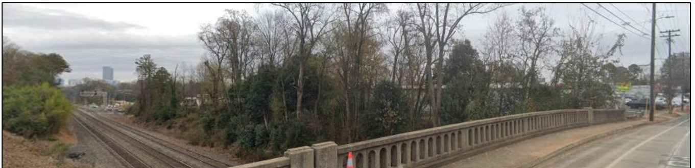
Street view of the site as seen from the Remount Road bridge over the Southern Railway line.
