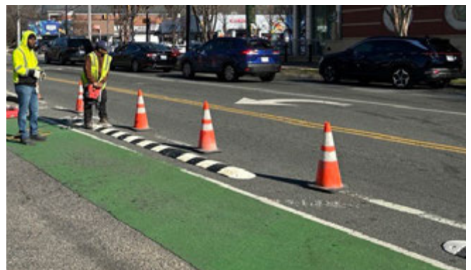
Image: CDOT crews installing vertical elements along The Plaza as part of the evaluation.
