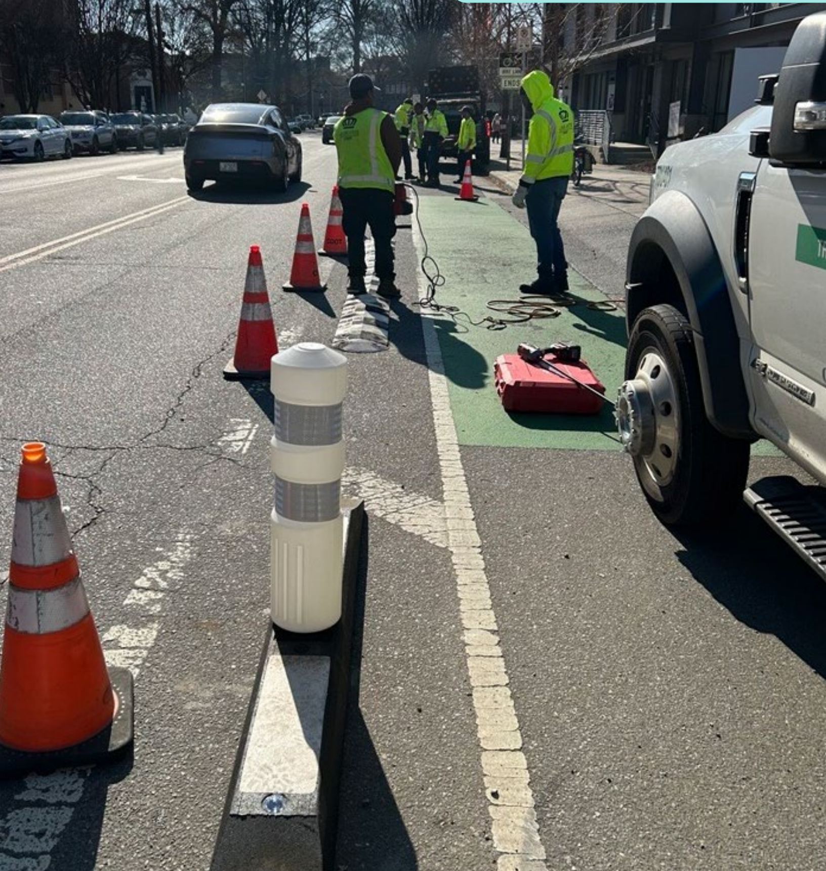
Image: A CDOT crew installs new vertical elements as part of an ongoing evaluation, testing treatments before wider deployment.
