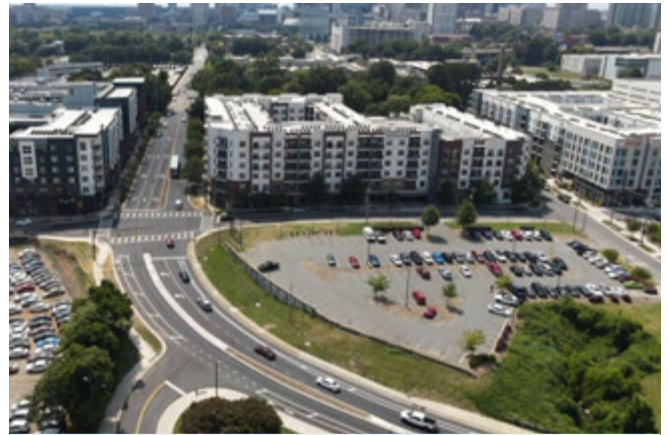
Image: Parkwood Avenue Streetscape.
