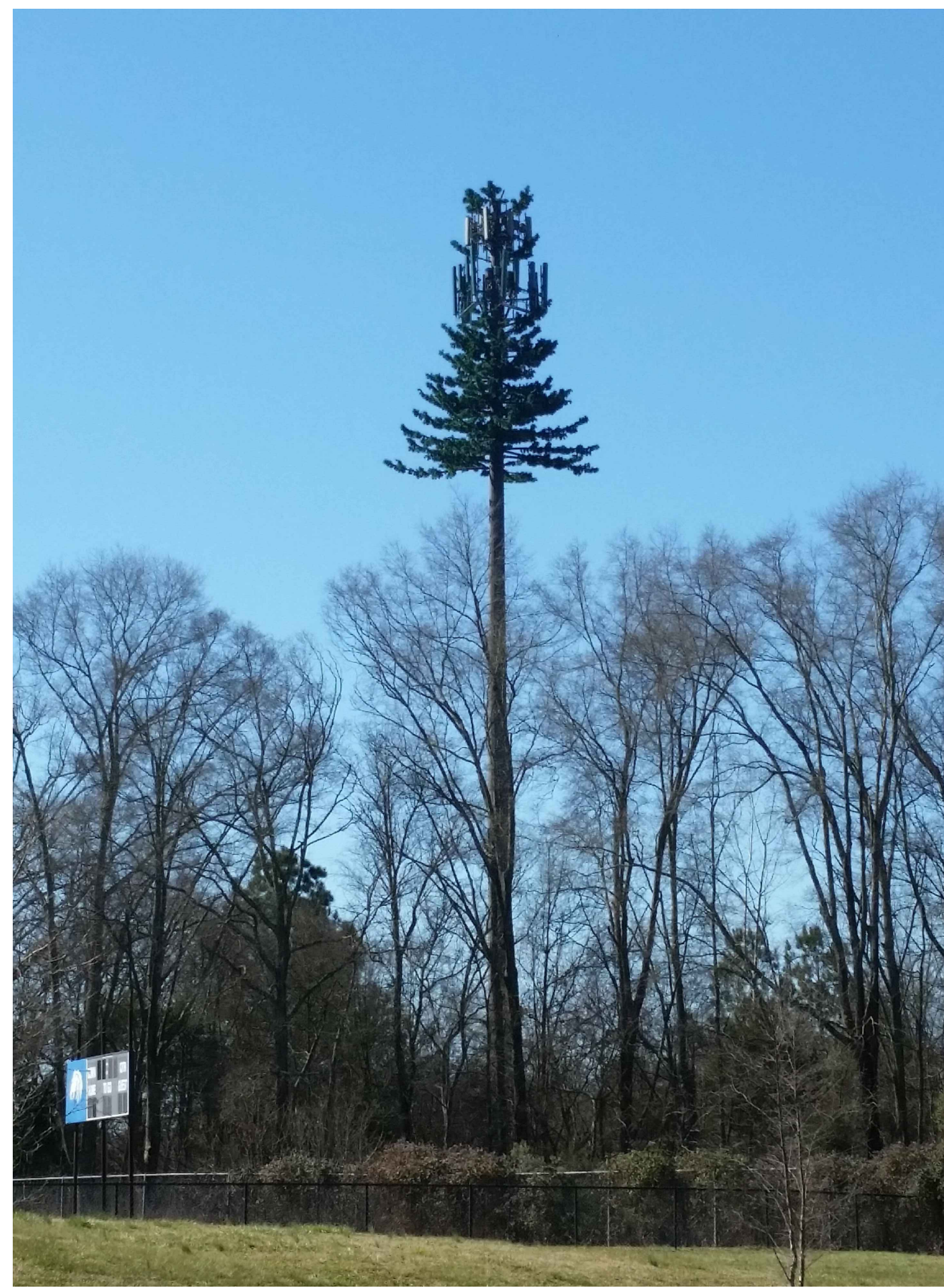
EXISTING COMMUNICATIONS TOWER STEALTH
