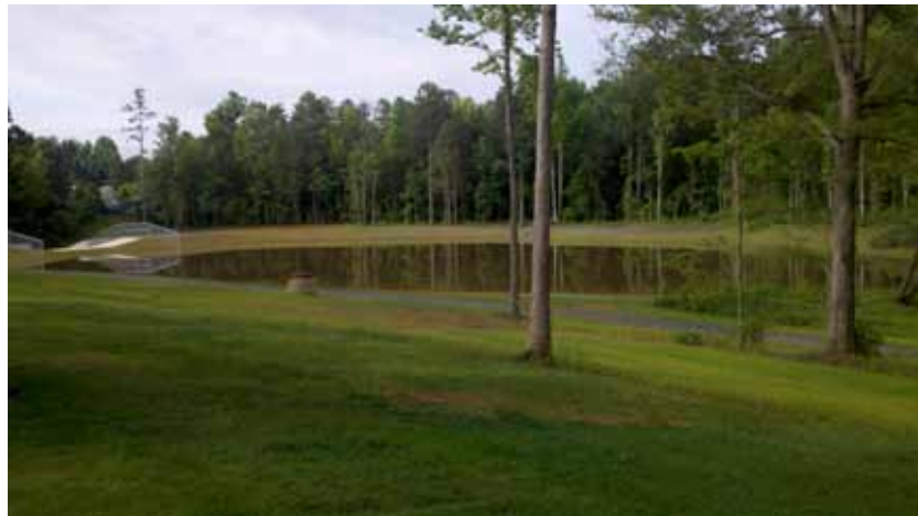
Stormwater detention ponds detain storm water and release it at a slower rate into storm drains, streams, rivers and lakes. This can reduce the risk of erosion and some flooding.
