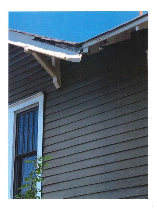
Replacing all rotten facia boards around the house using the same type of board that is currently used on the house.
