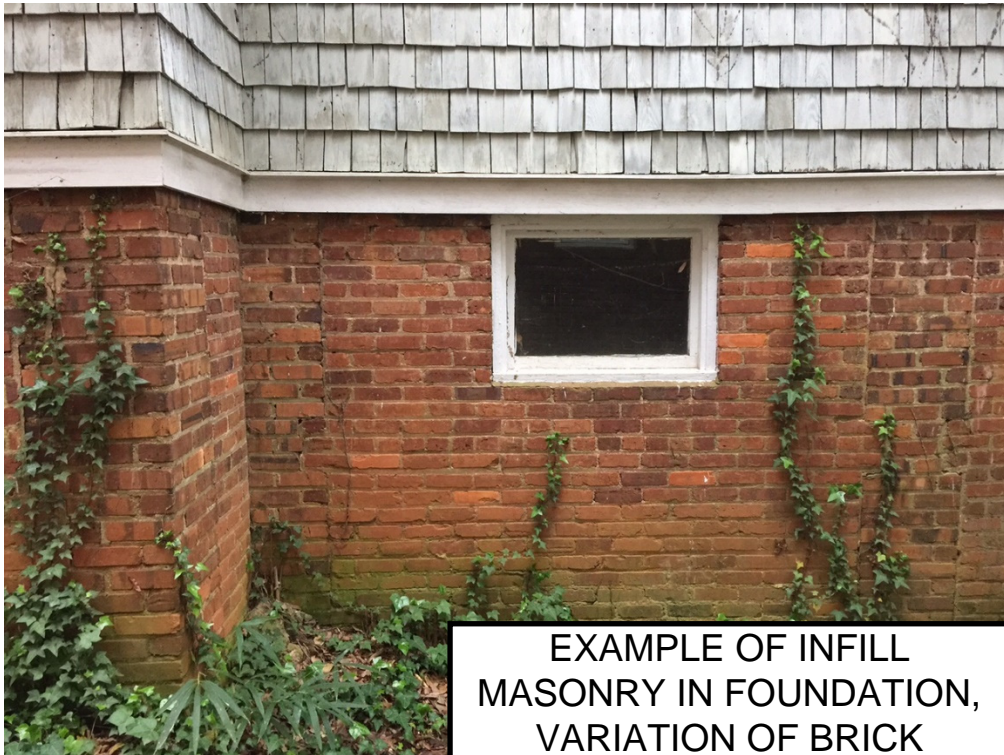
EXAMPLE OF INFILL MASONRY IN FOUNDATION, VARIATION OF BRICK
