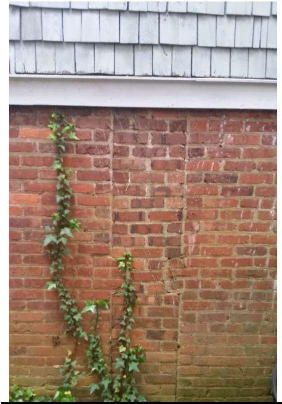
EXAMPLE OF INFILL MASONRY IN FOUNDATION, VARIATION OF BRICK
