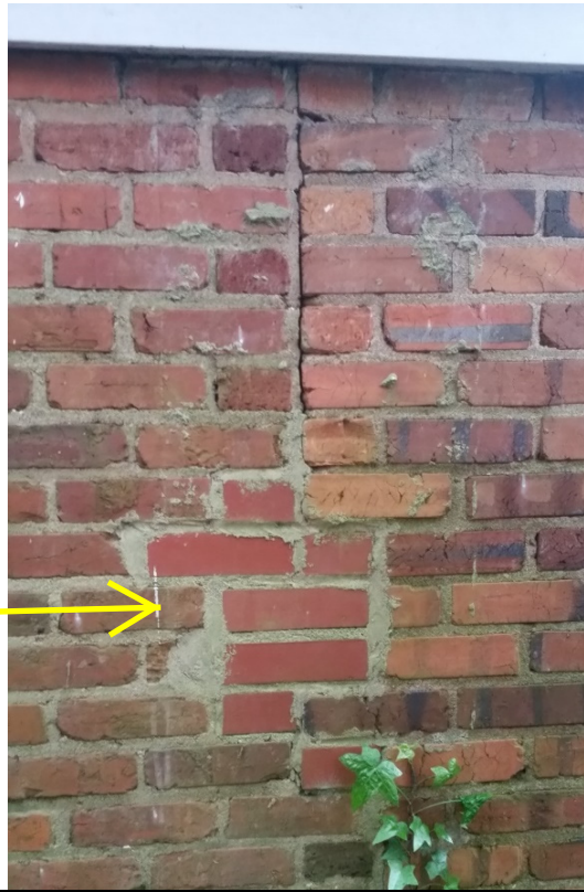
EXAMPLE OF INFILL MASONRY IN FOUNDATION, VARIATION OF BRICK
