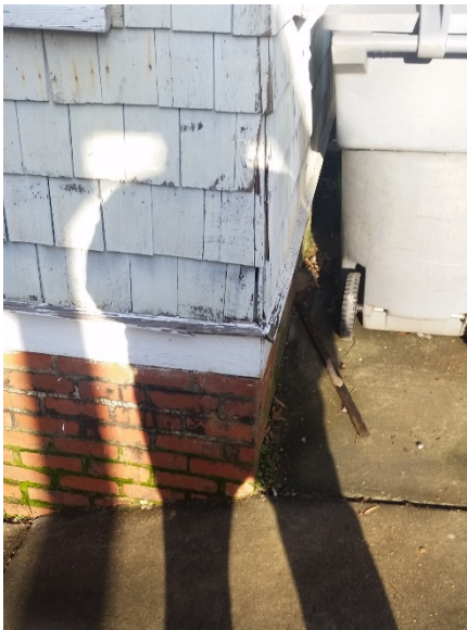
CORNER OF FOUNDATION OF ENCLOSED PORCH (DETERIORATION OF FOUNDATION AND WOOD BAND)
