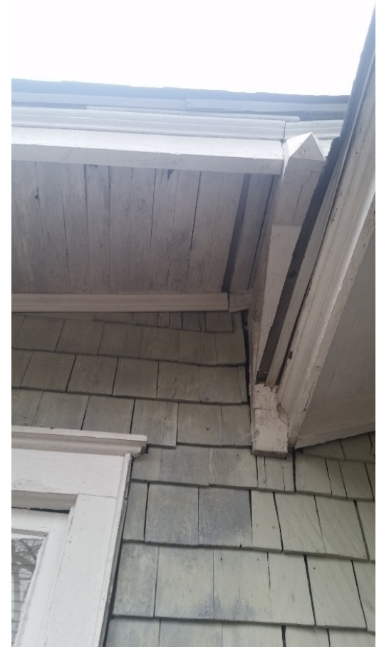
SIDE ENCLOSED PORCH AT ROOF, WALL IS SEPARATING
