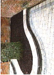
EXAMPLE OF HOW SMALL SUPPORT "WALL" WILL BE CONSTRUCTED (APPROX 6 INCHES OF HEIGHT TO ACCOMMODATE SLIGHT CHANGE IN LOT GRADE)
