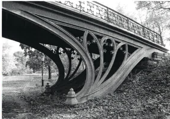
Cast-iron gothic tracery supports a bridge by Calvert Vaux, Central Park, New York City.
