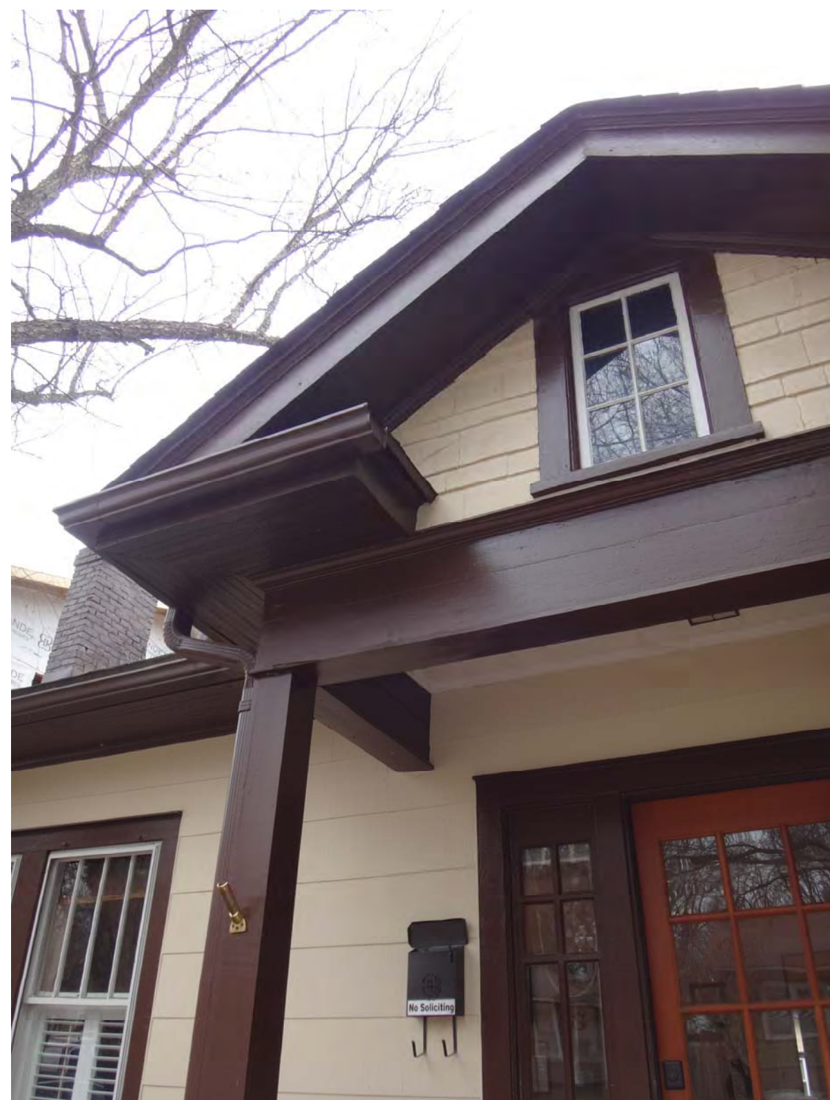
EXISTING RAKE-EAVE DETAILS
