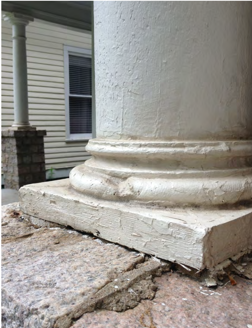
1 Existing Column Base Condition (typ.) A-1.1 1/4" = 1'-0"
