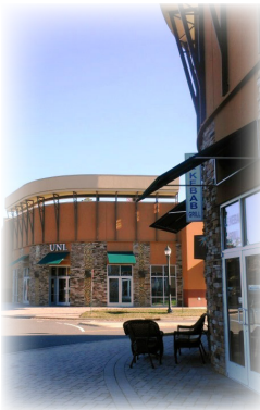
Grand Promande Village on McCullough Drive has both ground floor and second story retail spaces.
