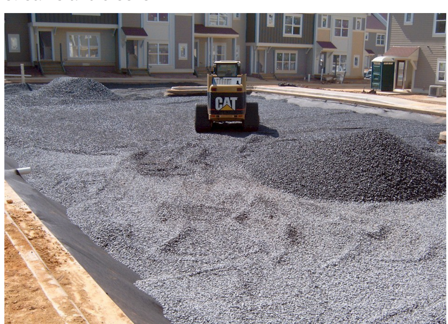
2.05 A pervious pavement parking lot is being installed to serve a multi-family residential development.
