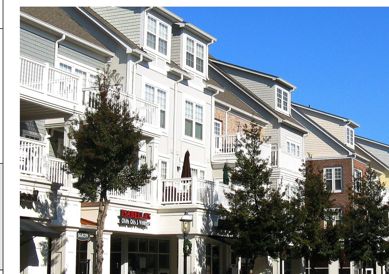
1.27 Variations in roofline and pitch work with small building components to reduce the perceived height and mass of this mixed-use center.
