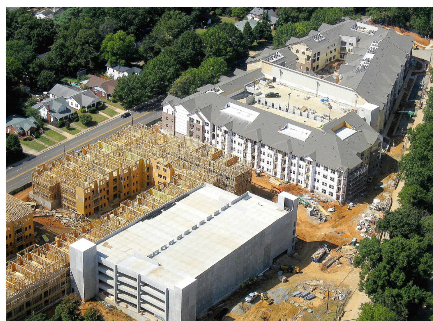
1.21 The parking structure incorporated into this multi-family residential development (under construction) reduces the surface area needed for vehicles.
