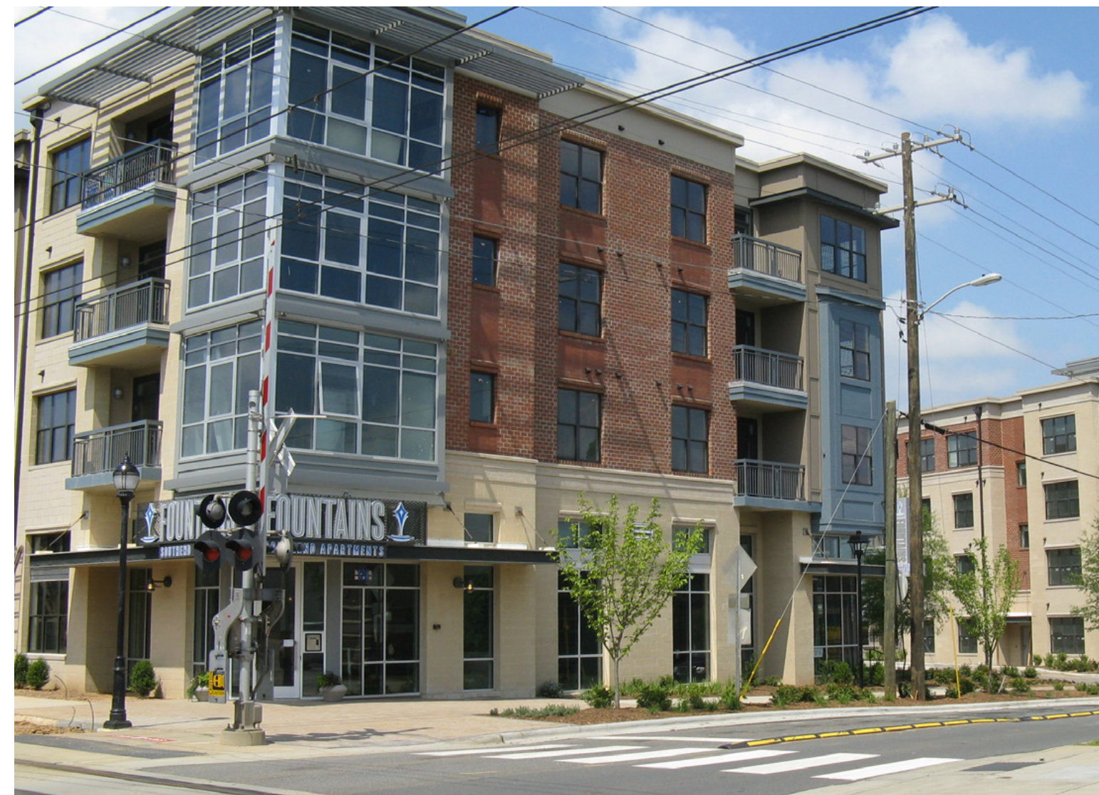
1.32 This ground floor of this multi-family residential building is visually distinguished from upper floors with larger openings and greater floor height.
