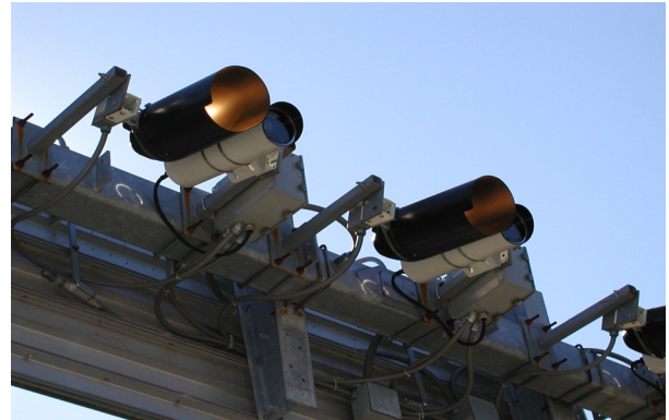
Figure 4: Electronic Toll Technology Applied to Managed Lanes
