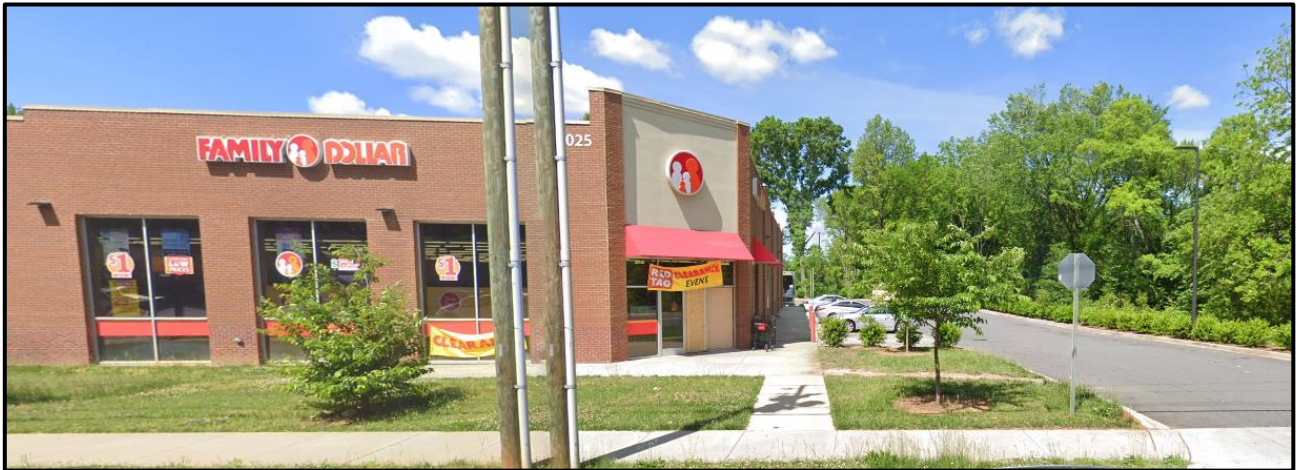
The property to the south along West Sugar Creek Road is developed with a Family Dollar store.
