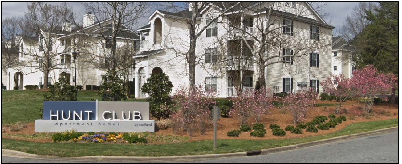
The property to the south and west along Northbend Drive is developed with multi-family apartments.
