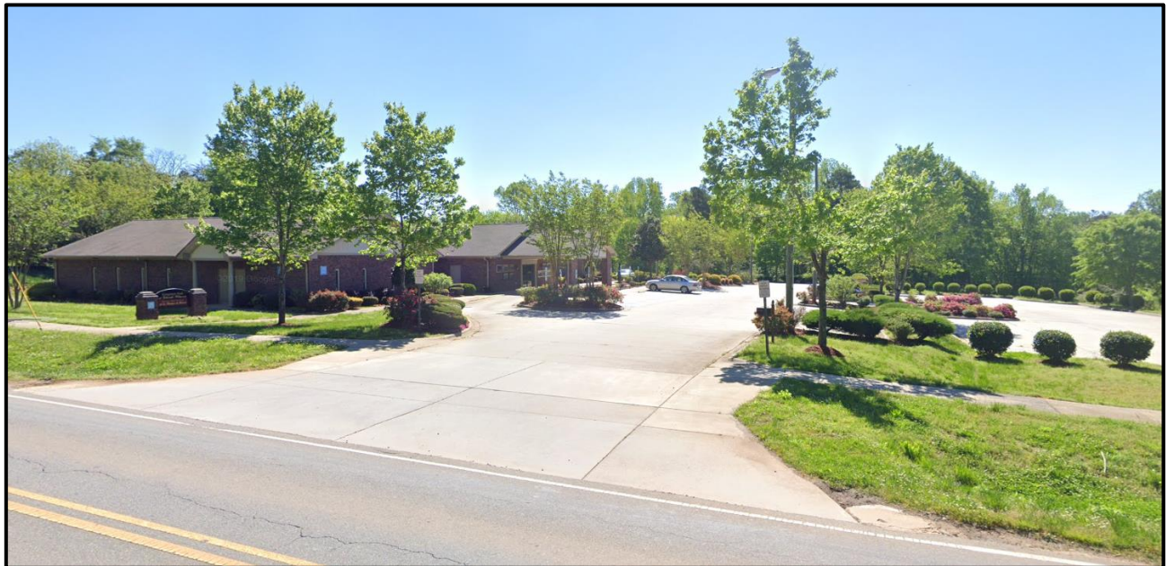
Facing away from site looking south toward institutional land use.
