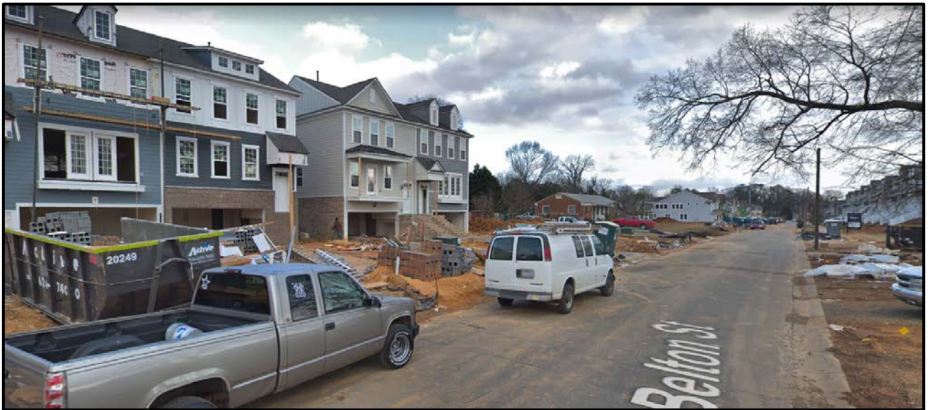
East are single family attached (townhome) units existing and under construction.
