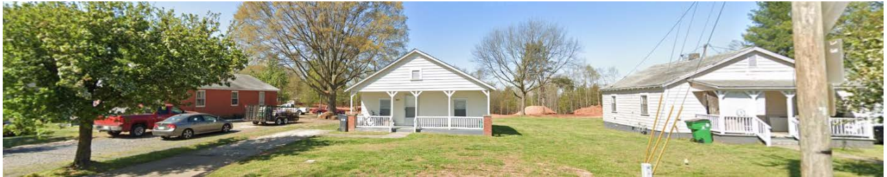
South of the site along China Grove Church Rd are single family homes.
