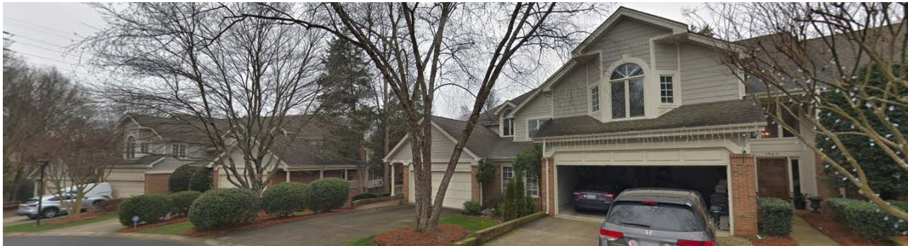
North of the site, across McMullen Creek, are single family attached dwellings along Meadowood Lane.
