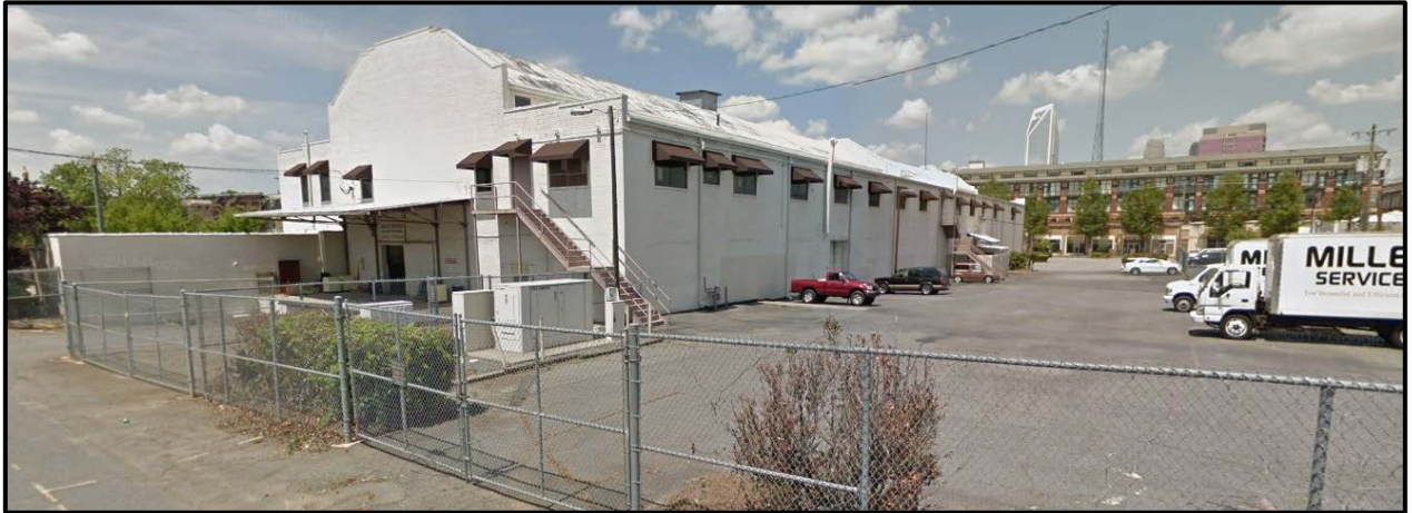
The property to the north along East Kingston is developed with a warehouse use.
