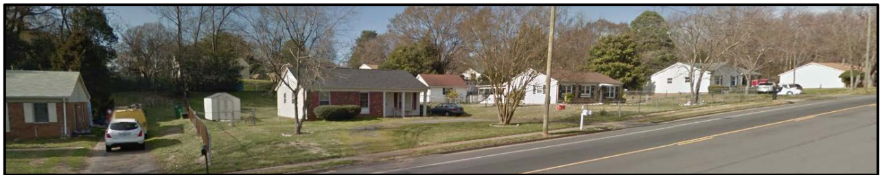
North of the site, across Arrowood Road, are single family homes in R-4 (single family) zoning.
