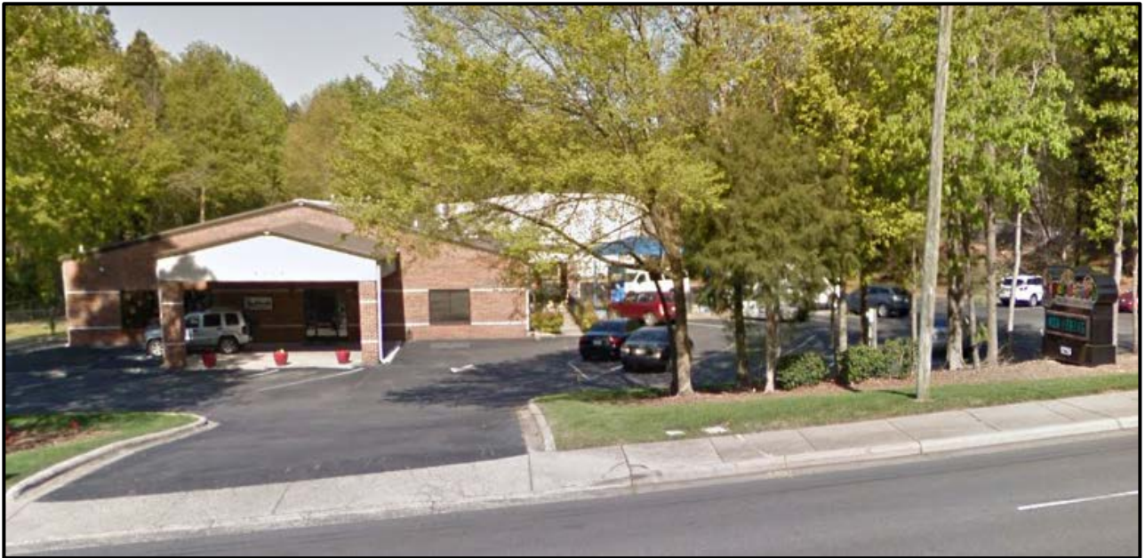
The subject property is developed with a daycare facility.
