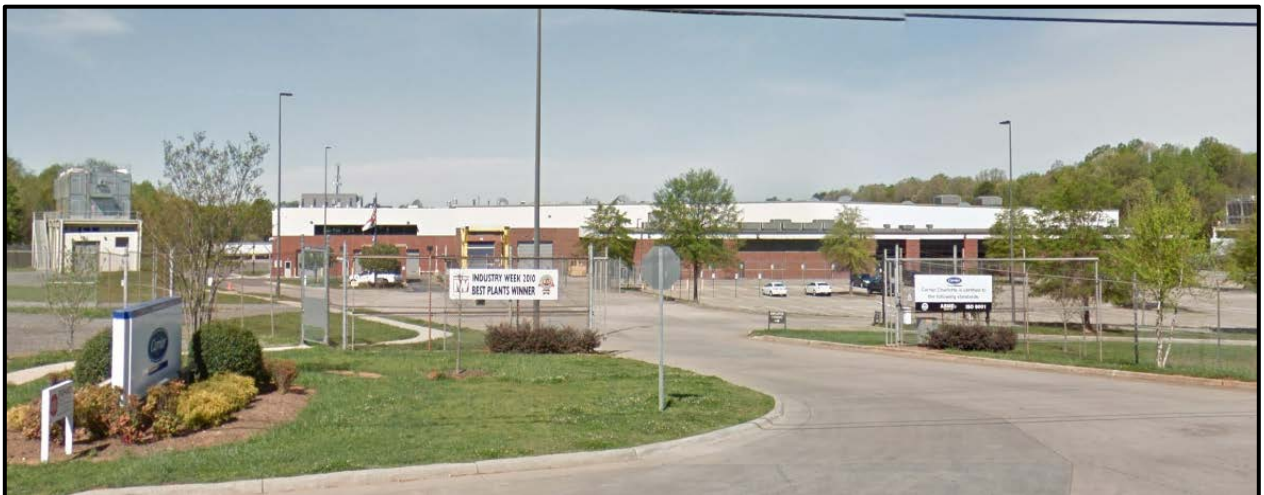
The property to the south along Old Statesville Road is developed with an industrial use.
