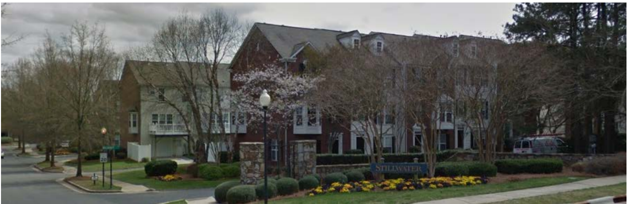
The property to the north and east along Elm Lane is developed with three-story single family attached dwellings.
