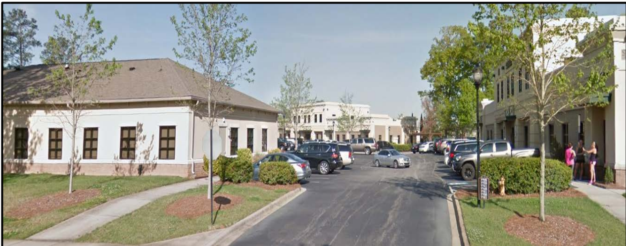
The property to the south along Williams Pond Lane is developed with an office park.
