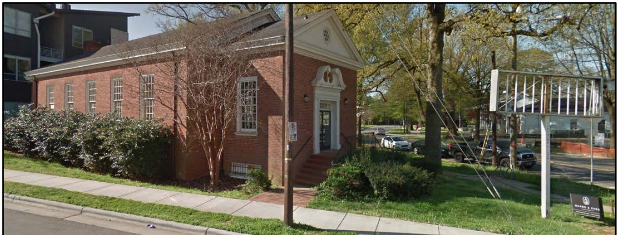
The subject property is developed with a church building that has been reused as a retail use.
