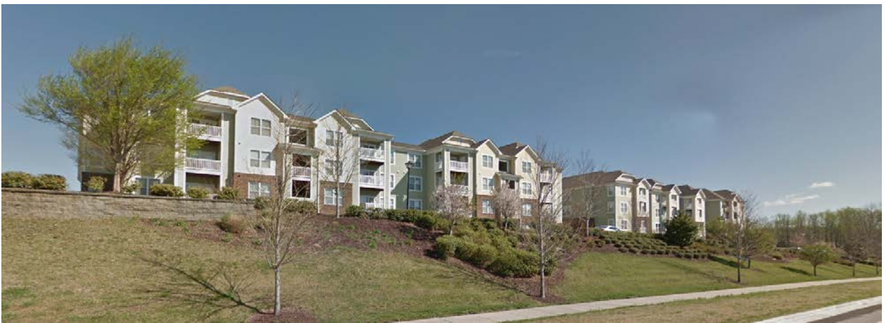
The properties to the north and east are developed with apartments.
