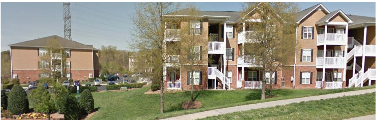
The property to the west is developed with apartments.
