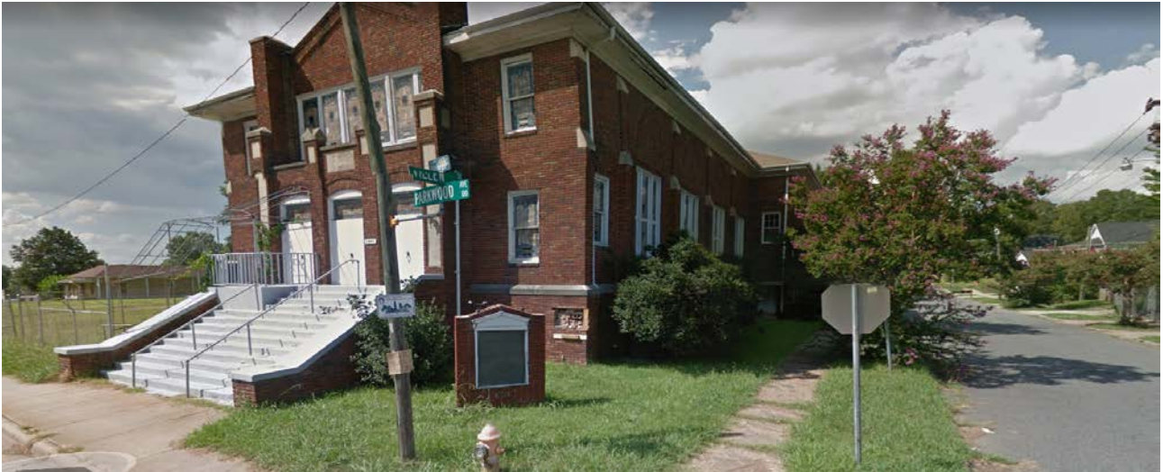
The subject property is zoned R-5 (single family residential) and developed with a former Church.
