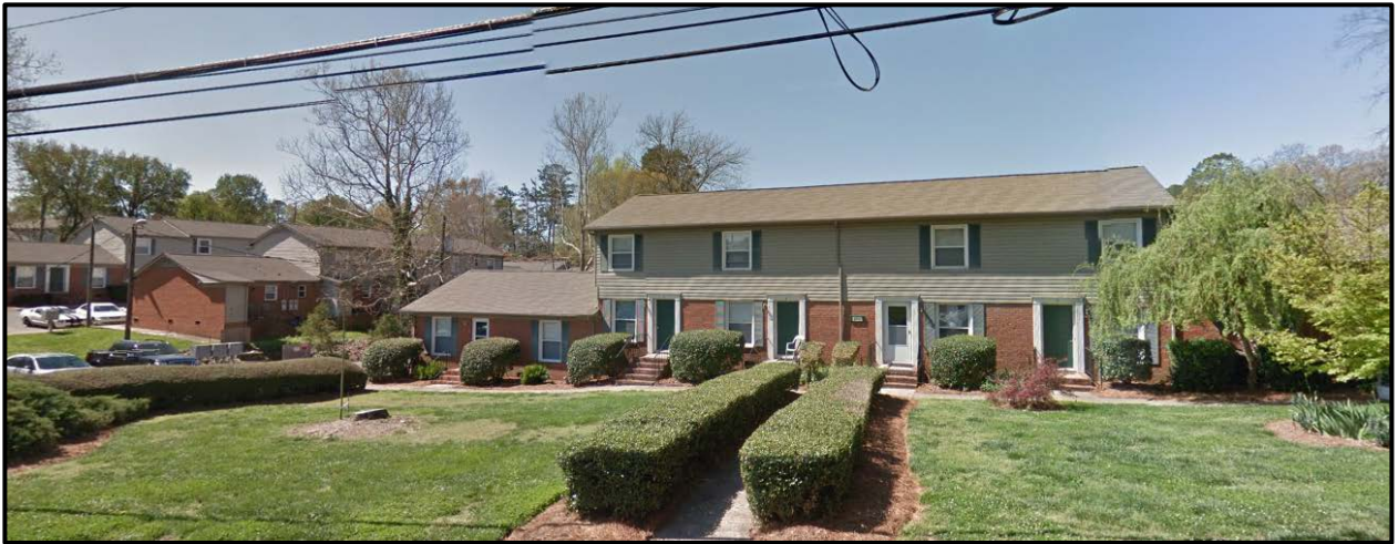
Properties to the west are developed with apartments along Craig Avenue.
