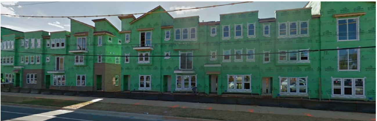
New apartments are under construction along Statesville Avenue to the south of the subject property.
