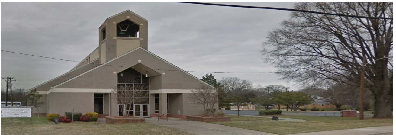
St. Luke Missionary Baptist Church is located across Statesville Avenue from subject property.
