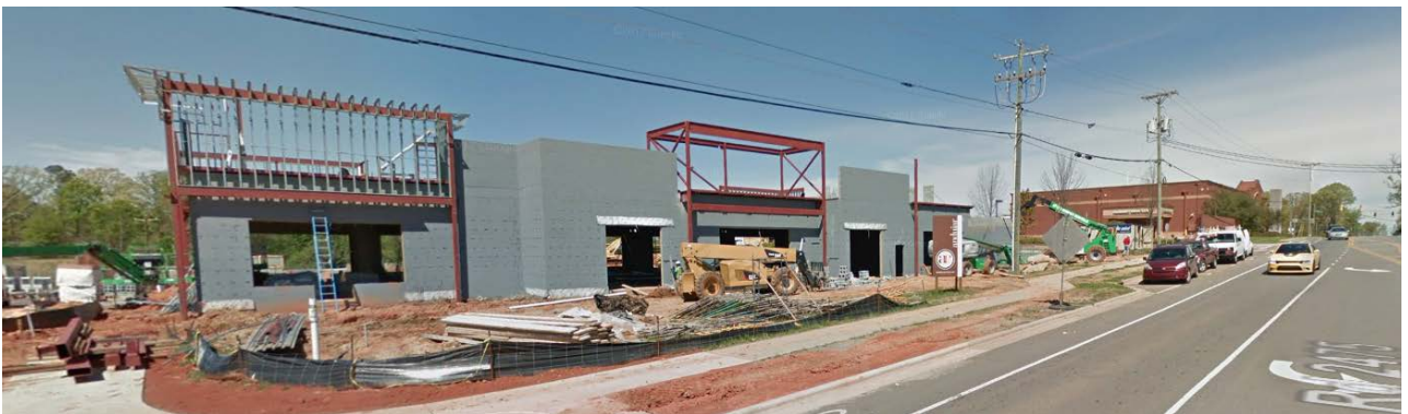
Property to the north is developed with a mixture of retail uses.
