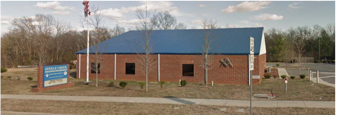
Steele Creek Masonic Lodge is located to the east.
