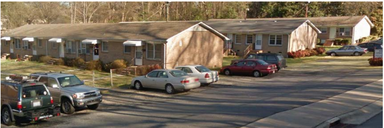
Properties to the north include multi-family and single family uses.
